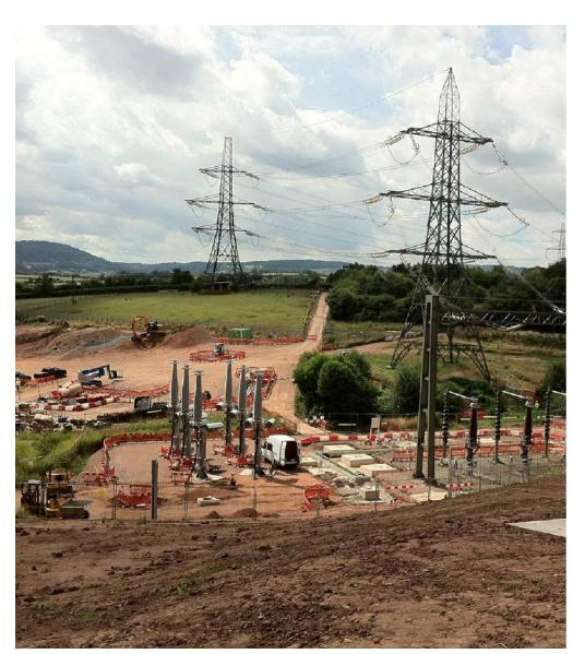
The undergrounding of electricity cables at Ross-on-Wye
